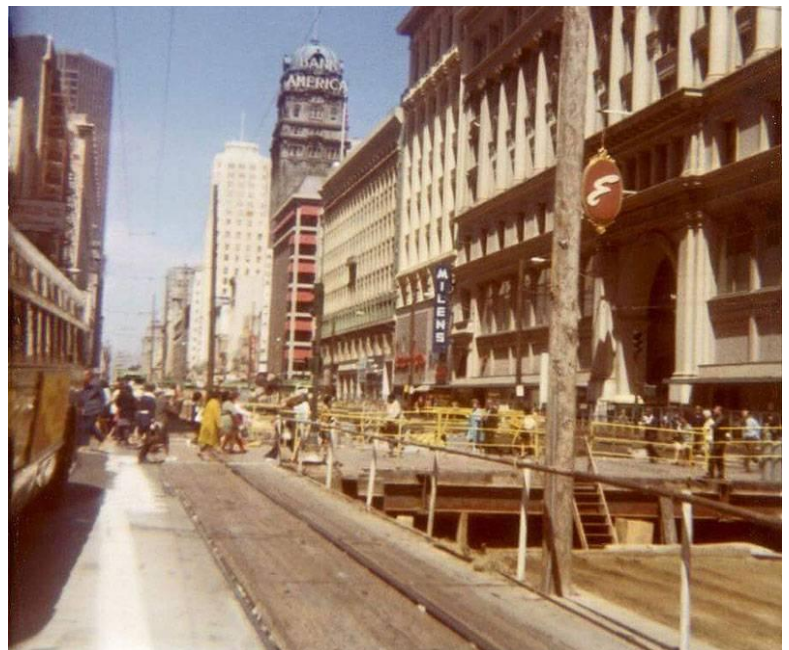
BART construction in 1960s along Market Street
